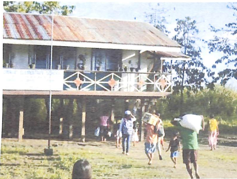
Two-classroom elementary school run by a local PO in Sitio Dinagat Photo taken: 02 April 2012
