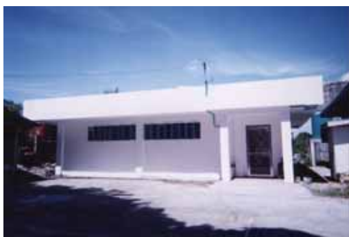
Handicap International's Rehabilitation Center in Cotabato City
