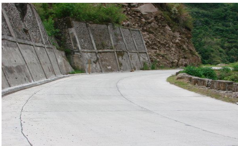
Figure 6. Portland Cement Concrete
