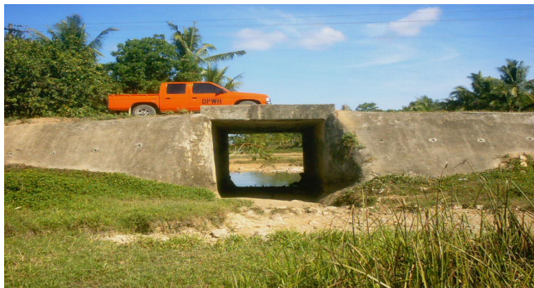
Figure 13. Animal Passage Culvert
