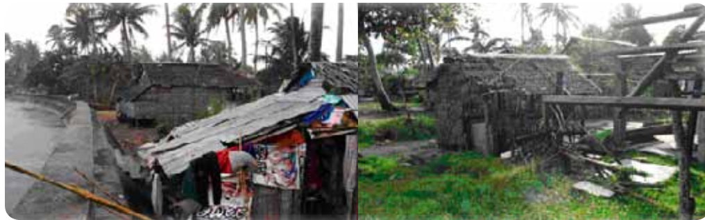
Fisherfolk's houses situated behind the seawall in Bagacay (left). Typhoon-damaged houses (right). The municipal government of Gubat has established an evacuation center on higher ground to shelter affected families. / Photos by UP-MSI.
