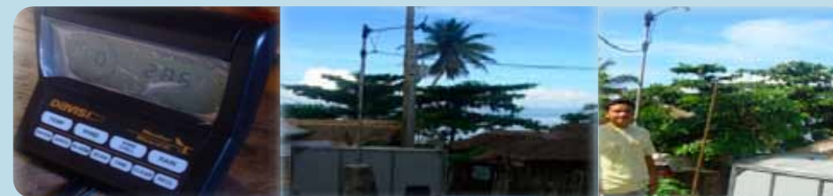
From left: The local weather instruments (wind vane, rain gauge, and Wizard 3) installed atop the residence of the weather monitor, J Sese in Burgos /Photos by PFEC
