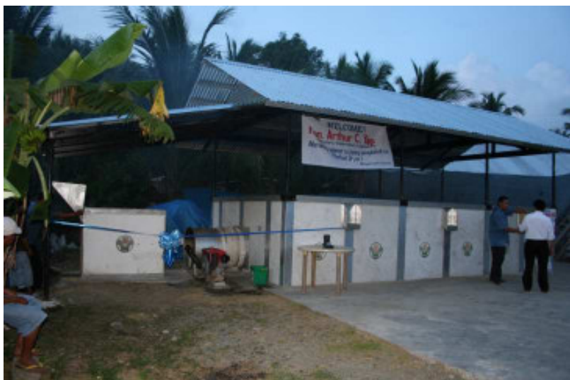
A typical DA-BPRE flatbed dryer.
