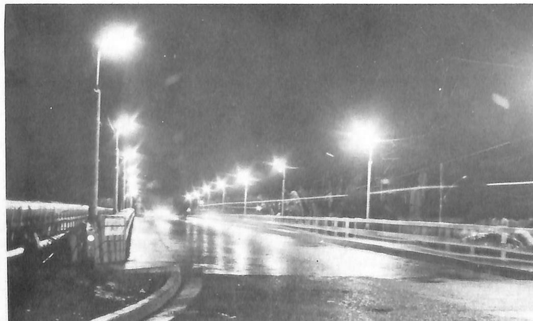
BANKEROHAN BRIDGE. — Since its implementation in September 1983, the program enabled the city government to save as much as 50% in electric bills. Under the street light program the maintenance and replacement costs of bulbs have been shouldered by the Davao Light and Power Co.
