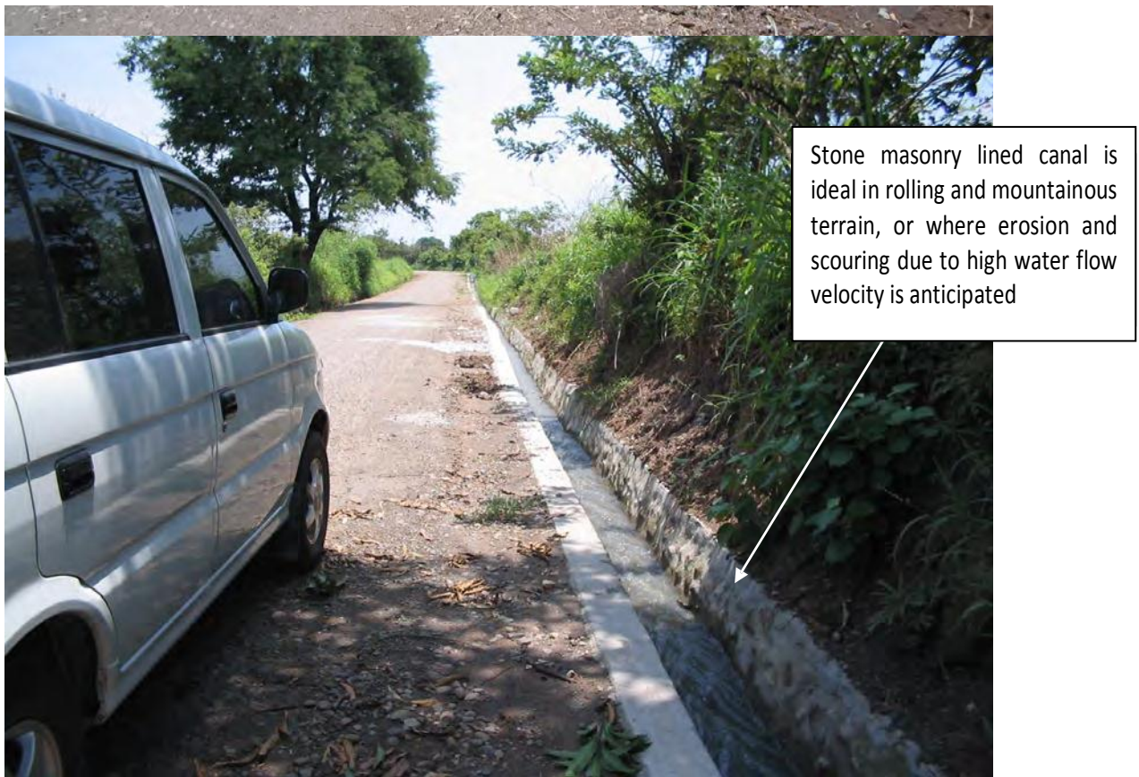
FMR with concrete/stone masonry lined canal. (ARCDP2)
