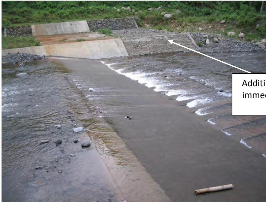
Slope protection built immediately upstream of the dam.
