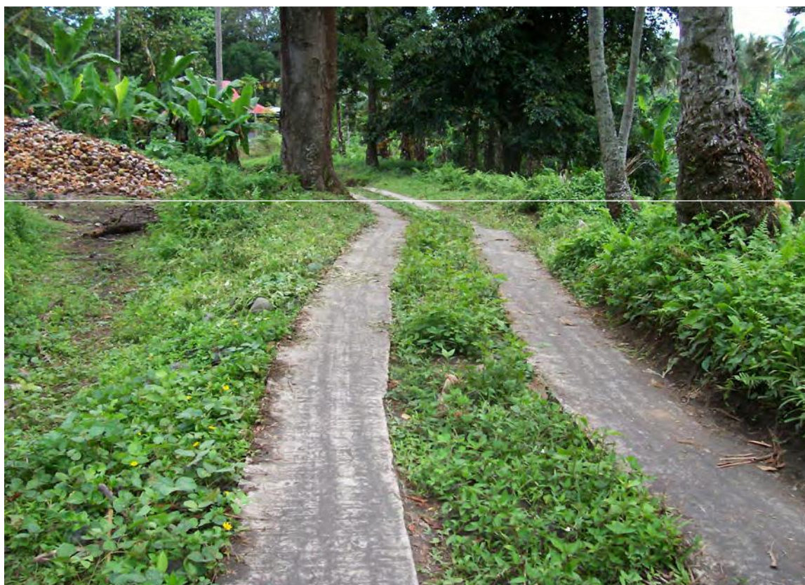
In some cases a concrete tire path may be a more practical alternative design for rural roads. (ASFP)
