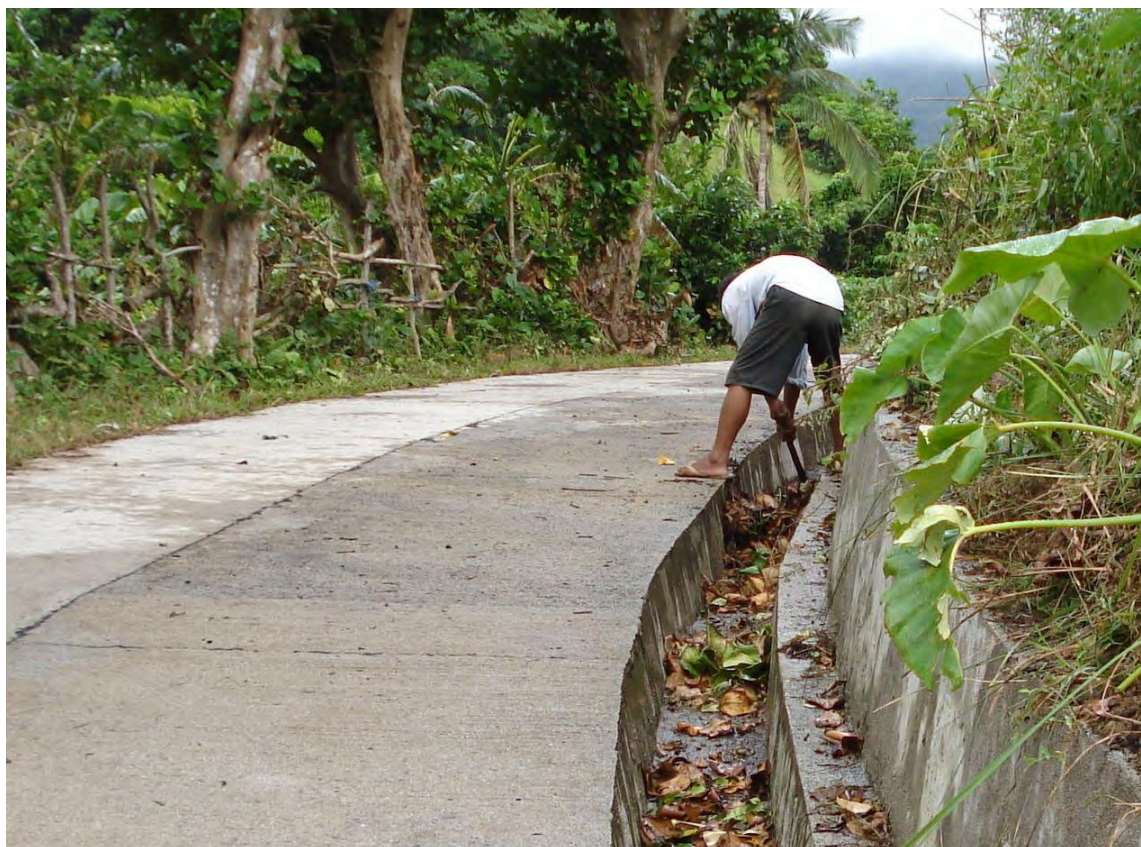
Shown above is a member of the local O&M group doing his share in cleaning the road's side canal. (ARCDP2)
