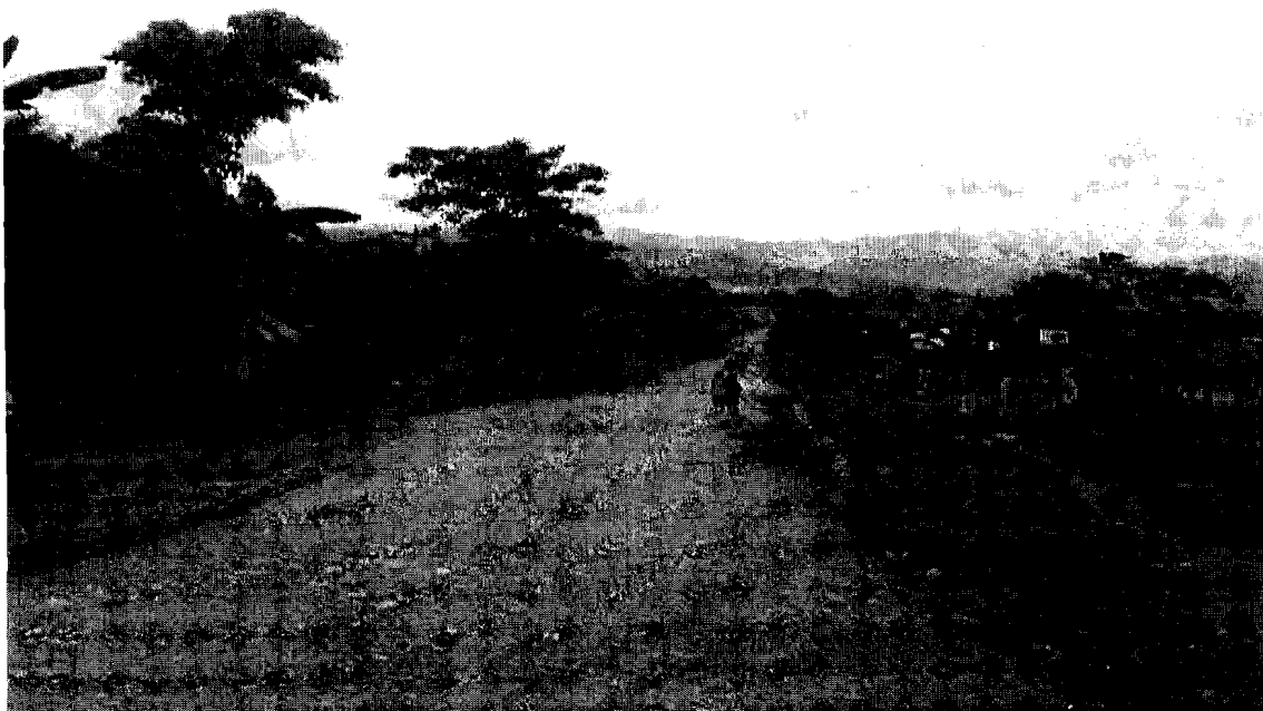
Existing Gravel Road @ Km. 180 + 800 Brgy. Nasucob
