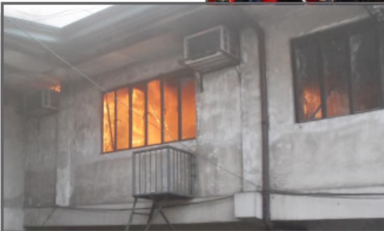
The July 20 fire, which lasted for almost two hours, tore down parts of the LDC and NAFC offices and resulted to P10M-worth of damages. Sec. Alcala who witnessed the raging fire, commended the united efforts of the BFP, QC fire department, Dear John janitorial services and other volunteers.
