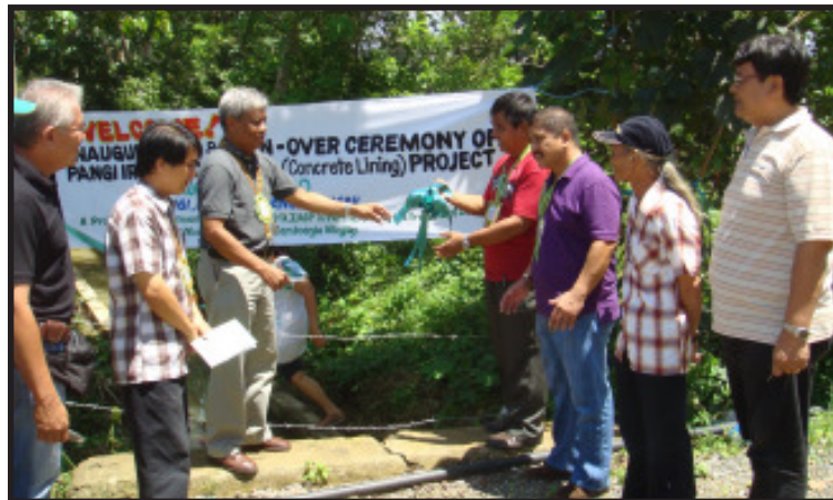
DA Region 9 Director Oscar O. Parawan (3rd from left) leads the inauguration of the P2-M canal concreting of the irrigation system in Upper Pangli, Ipil, Zamboanga Sibugay.
