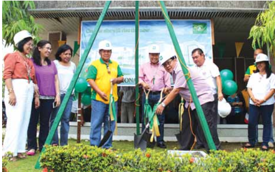
NEW NIA OFFICE BUILDINGS NIA Bicol Regional Director William P. Ragodon (foreground) shovels cement on the hole containing the time capsule of the new 2-storey NIA Regional Office Building that will replace the old building inside the agency's compound along Panganiban Drive, Naga City. Looking on are: (from right) Naga City Mayor John Bongat, NIA Administrator Antonio S. Nangel, and Silvestre Bonto, president of the Bicol Region Confederation of Irrigators Association. Others in photo are (from left): NIA PAIS Manager Pilipina Bermudez, Mrs. Arlene Ragodon, Ms. Merle Bongon, and NIA Albay-Catanduanes chief, Engr. Cristeta Mesias. Ragodon, Nangel, and Bongat likewise broke the grounds for the NIA Bicol Farmers Training Center within the NIA compound.
