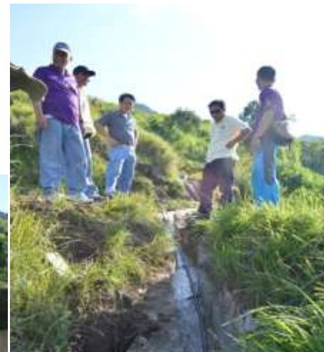
Rehabilitation of Challug-Mangay Communal Irrigation System in Bugnay, Tingalyan,
