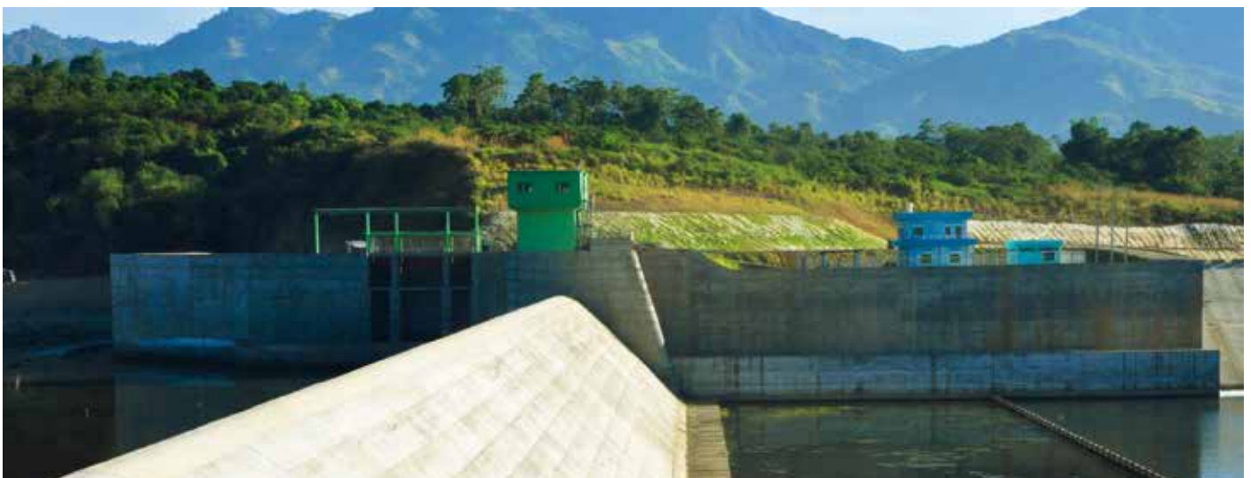
Agno River Integrated Irrigation Project (ARIIP) Re-regulating Pond
