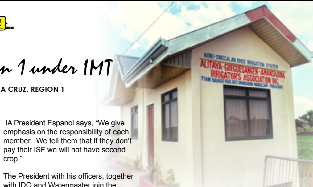
AGA IA Office (Constructed thru IA Incentives and donations from other offices)
