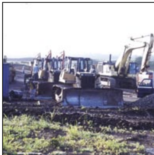
▲ Heavy equipment utilization in Bohol II Irrigation Project
