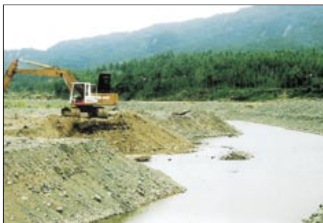
▲ River rechanneling at Agos RIS, Infanta Quezon, Region 4
