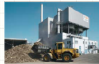
Biomass-fired CHP plant at Ilmenau
